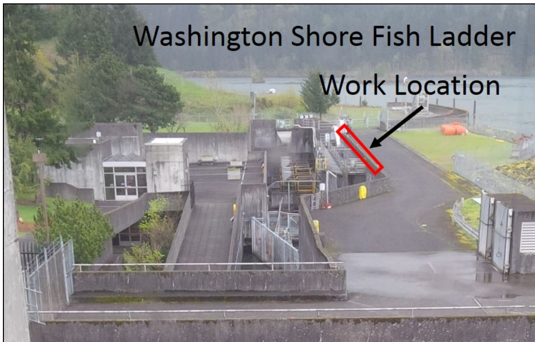
Figure 1. Bonneville Washington Shore Fish ladder exit. The location where new conduit will be installed to replace existing flow sensors.
